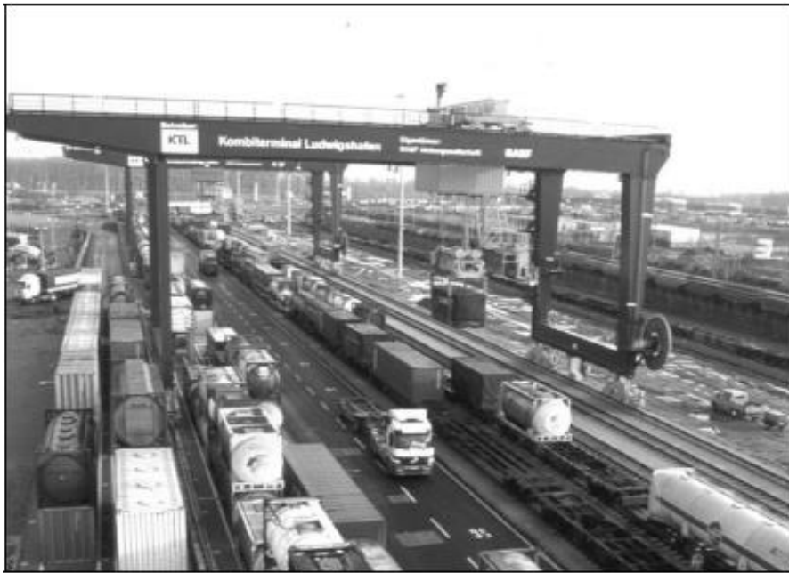
Figure 4. Example of a road-rail transport terminal.
